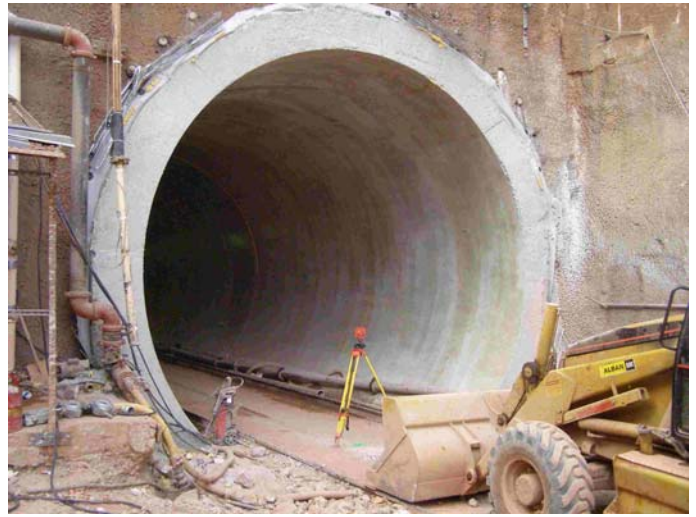
Figure 3. Finished Final Lining of East APM Tunnel
