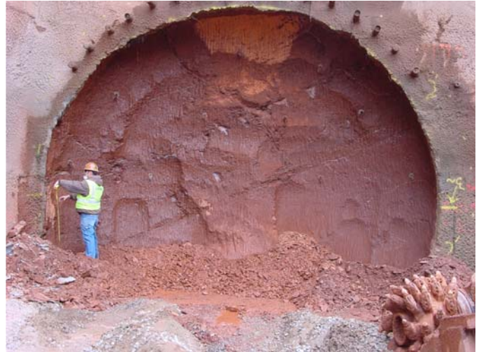
Figure 2. Typical Face Conditions
